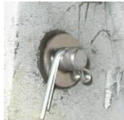
The end of the shaft with cotter pin is shown in next photo. After the pin was removed the shaft was free to slide to the left. The top of the shaft and the side of the control were marked so that the control lever can be reinstalled in the same position. The next task was to disconnect the control rod from the control lever, remove the spring attached to the control lever, slide the shaft towards the left and slip the washers off the end of the shaft.
