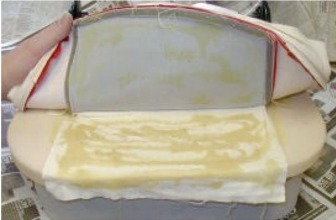
Next, the U shaped edge roll was cemented into place on the bottom foam over the cloth strips attached in the previous step as shown in next photo.
