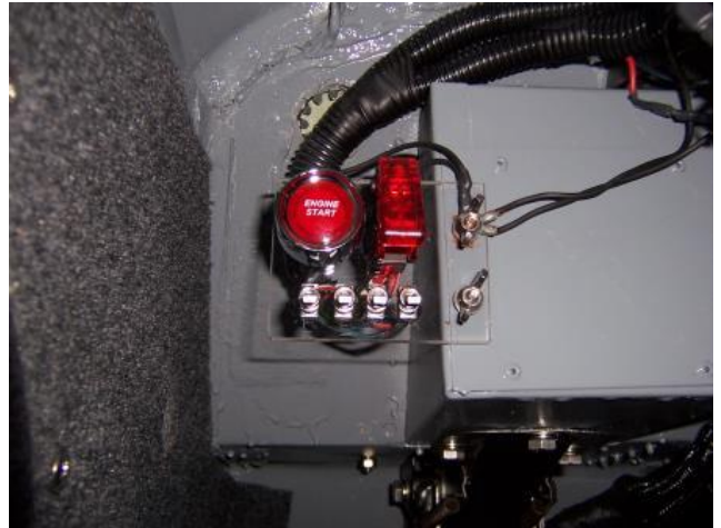
Switch Panel under the dash – very compact
