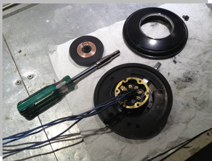
Putting a new wiring harness on the control head
