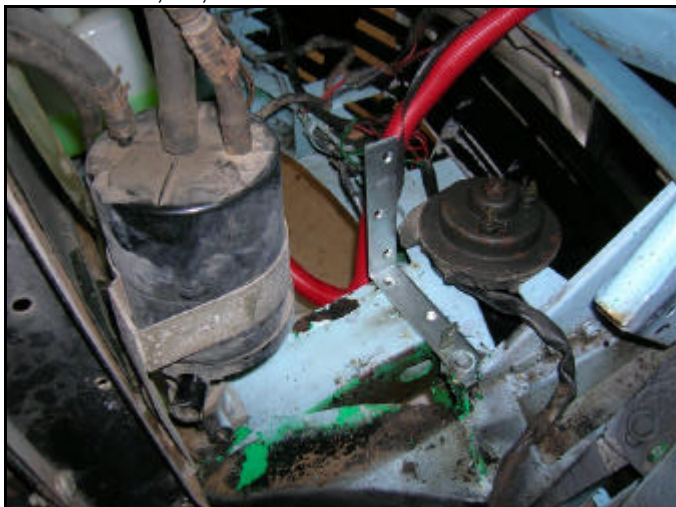
Filter assy. With lower hose removed for deflector installation. Second large L bracket for new lights.
