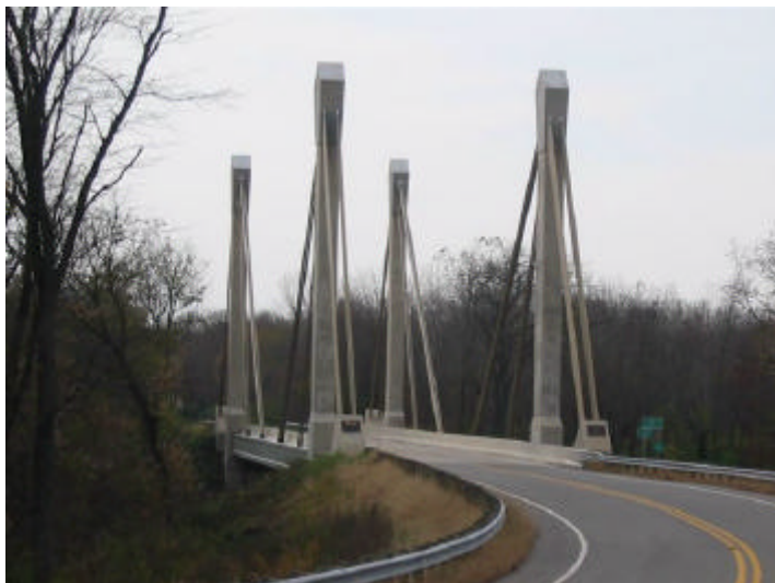
Cool 'cable stay' bridge crossing Big Darby Creek
