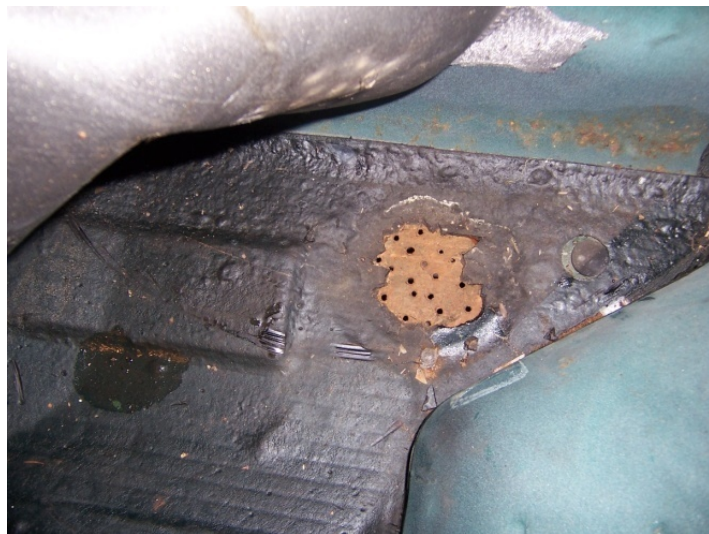
Remember – if you can't wait for rust to make the drain hole, use an awl!
