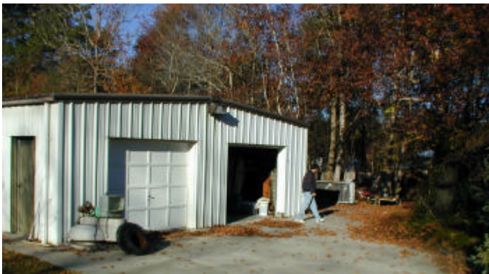
Ed’s “Shop” (I want this building)
