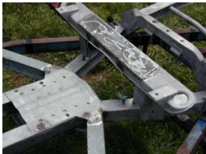
All of the reinforcements have been done.
