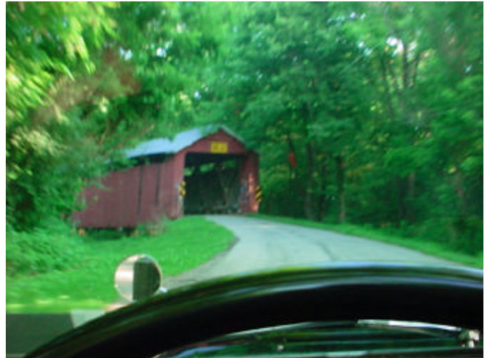
Saturday EMR - Charleton Road Bridge – The Approach From The Leader Of The Pack
