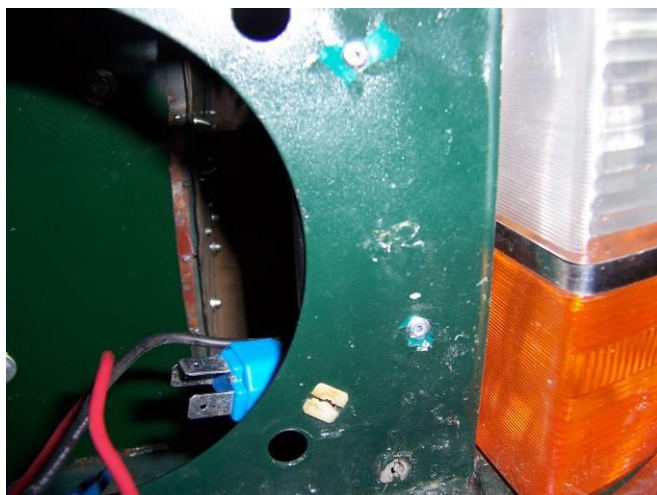
Driver's LED Power Converter Pop-riveted to back side of the front valence, driver's side. Evidently the paint here wasn't prepped good for that last respray....
