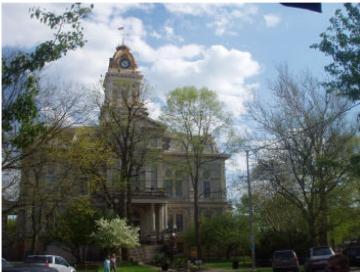
View of the Courthouse from the Midland - what a perfect day "weatherwise"
